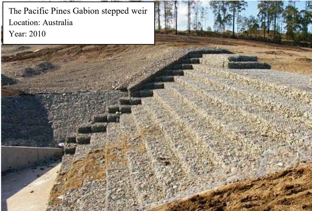
**Figure 1-9.** Gabion stepped weir, Pacific Pines, Australia, 2010
