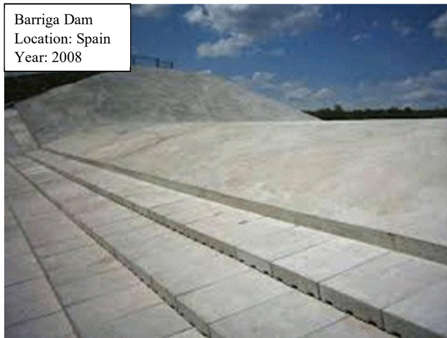
**Figure 1-16.** Pre-cast concrete with overlapping, Barriga Dam, Spain, 2008
