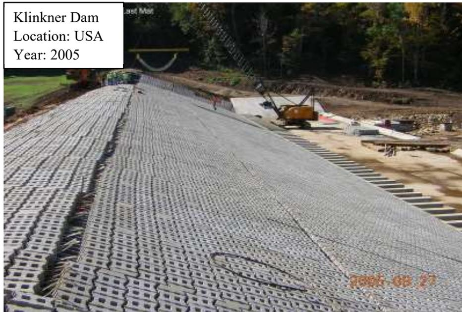
**Figure 1-15.** Pre-cast concrete without overlapping, Klinkner Dam, USA, 2005
