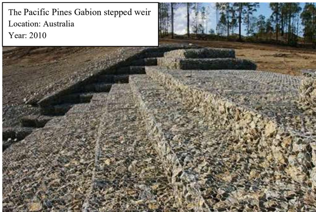
**Figure 1-10.** Gabion stepped weir, Pacific Pines, Australia, 2010
