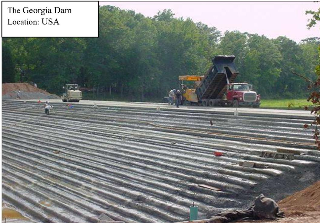
**Figure 1-12.** Site-cast concrete, Georgia Dam, USA
