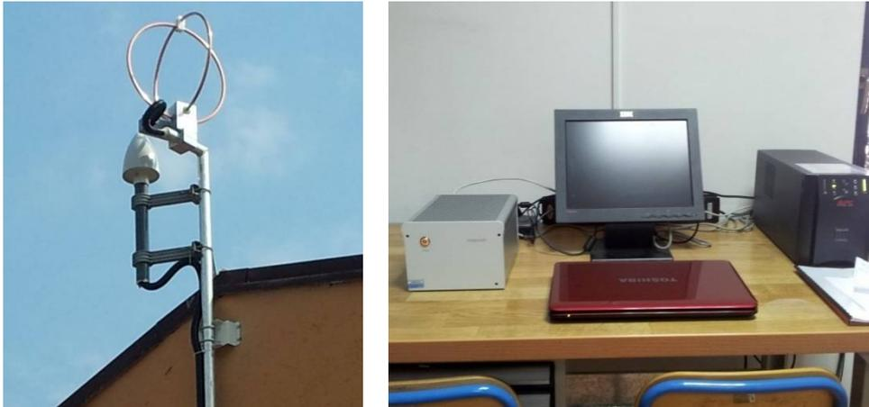
Figure 4.2.3. LINET sensor installation
