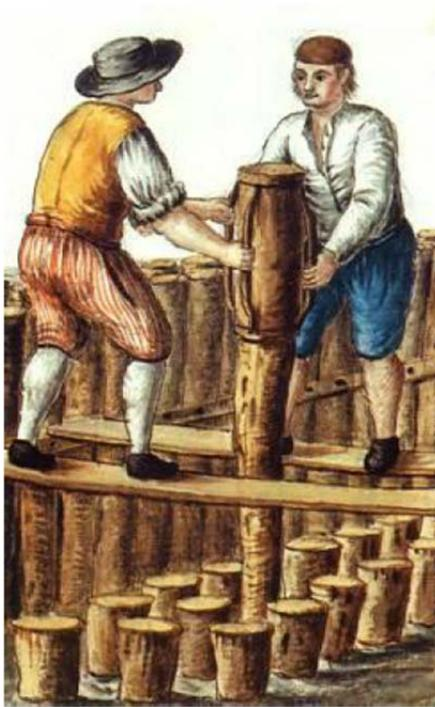
Figure 4: Watercolour by Grevembroch, G. (18<sup>th</sup> century), which illustrates two workers driving wooden piles into the subsoil using a *battipalo* [see Trovò (2012)]
